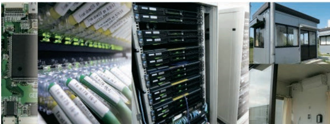
VLSI and embedded systems, network devices, servers, and smart house experimental environment
